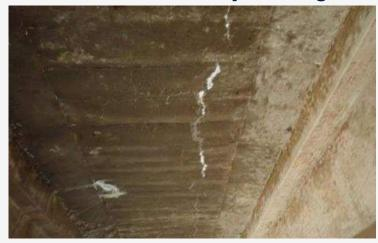
Longitudinal cracks with efflorescence in underside of deck between beams.
