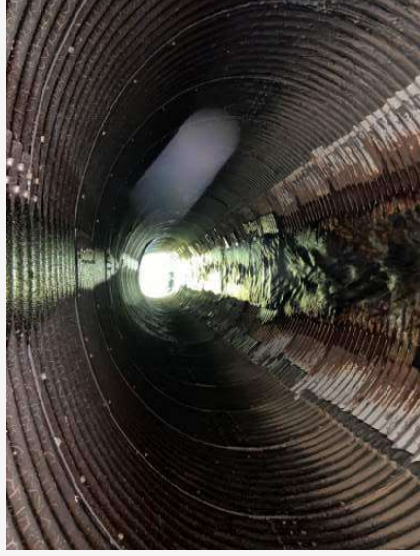
Culvert – Towards outlet
