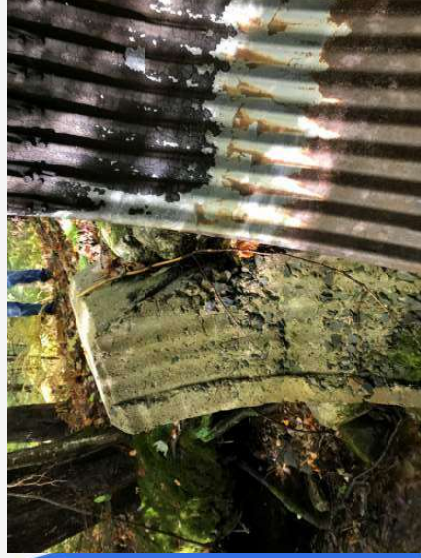
Pipe condition (perforation)
