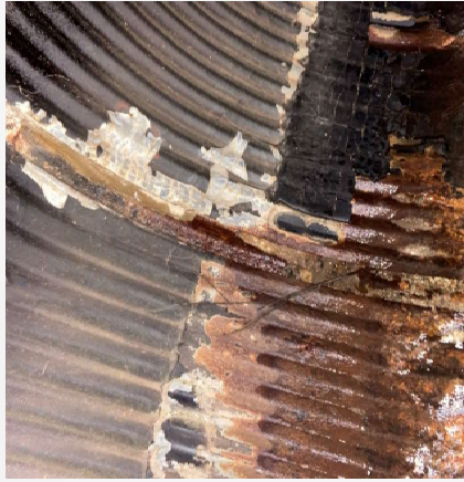
Pipe condition (perforation)
