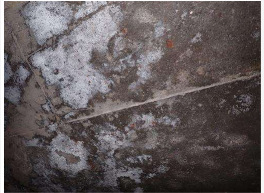
Underside of west slab edge with frosting
