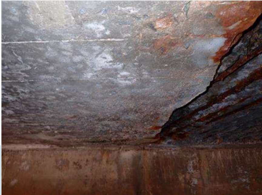
Large hollow and scaled area underside of slab
