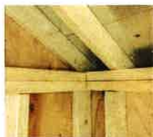
Double top plates are used on all 4 walls except on Mini-Barn and Townhouse sheds.
