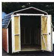
Doors are reinforced with 2" x 4" bracing.
